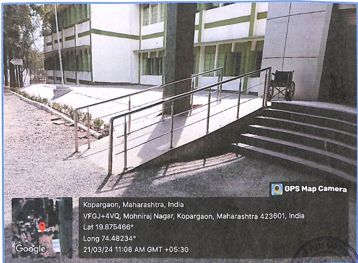
Ramp and Rail at College Main Buliding
