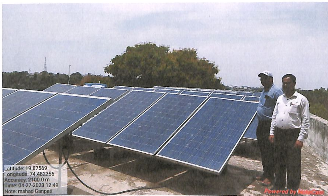
10KW Solar PV system installed on roof top of Library Building.
