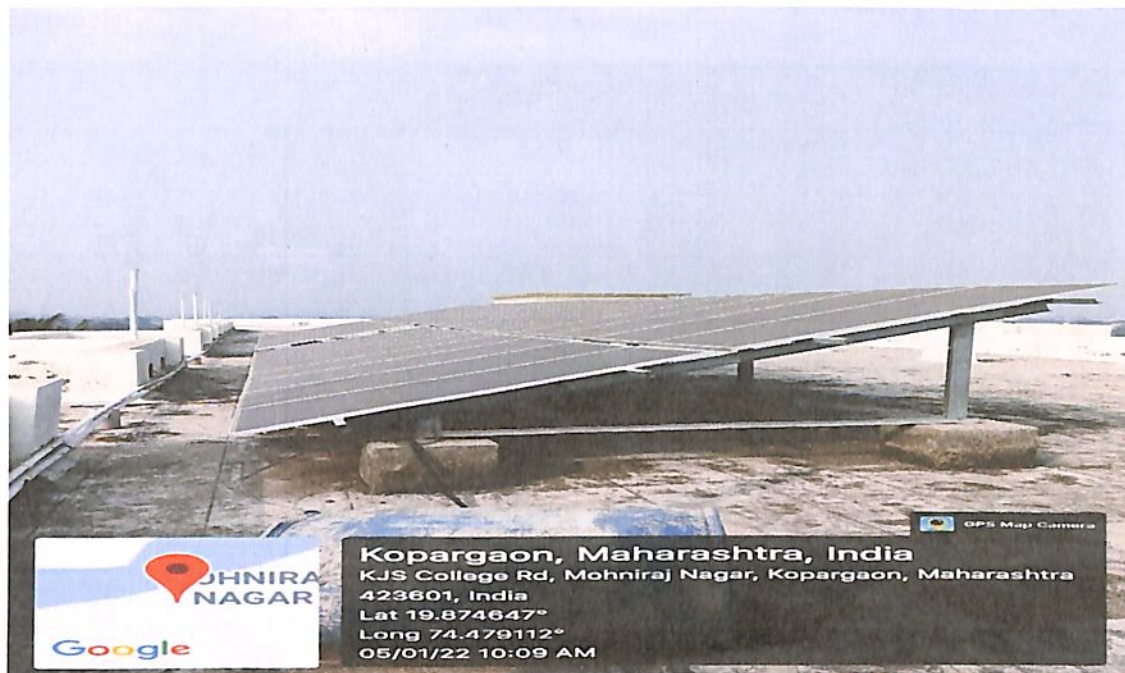
10KW Solar PV system installed on roof top of Science and Technology building.
